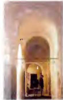
Ribs of the tunnel vaults of the Ribat of Susa, built in 821–822 CE.
